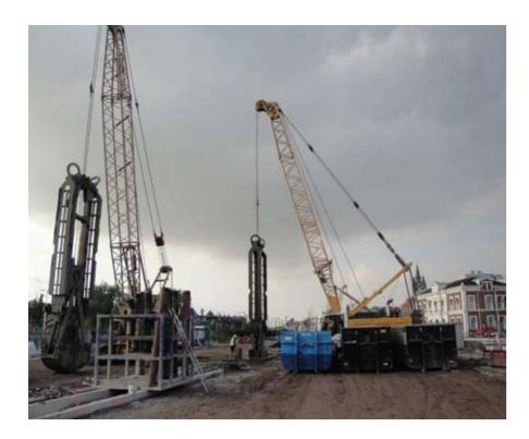
If a tunnel, building excavation or underground parking station is to be constructed in an urban area, diaphragm walls are in many cases an attractive option. These concrete walls are placed in a trench in the ground. The advantage in densely populated areas is that no vibrations are produced when the walls are put in place. Diaphragm walls can also support large vertical loads. INTRON consultant Michel Boutz was involved in three such projects over the past six months.
