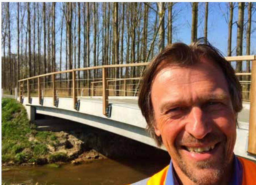
Martin Verweij at the bicycle bridge near Valkenswaard in The Netherlands, made of geopolymer concrete with the binding agent SQAPE
